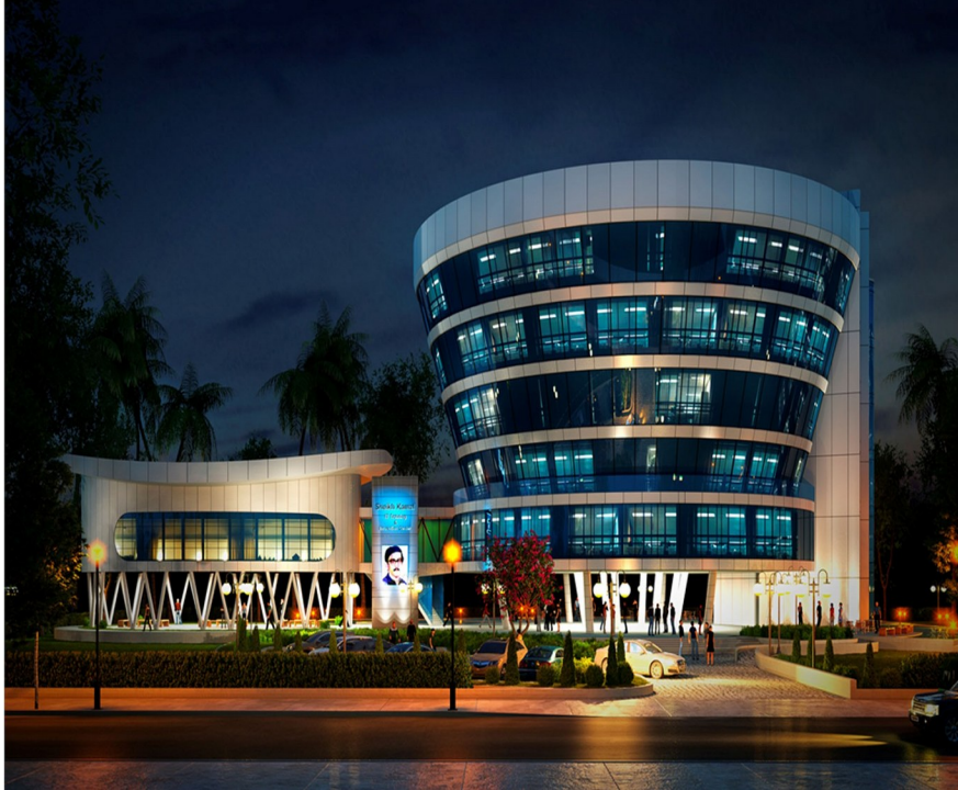
Design of the IT Parks in 7 District (Construction ongoing)
